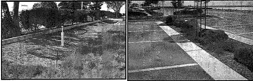
Figure 5.4. Infiltration Trenches
